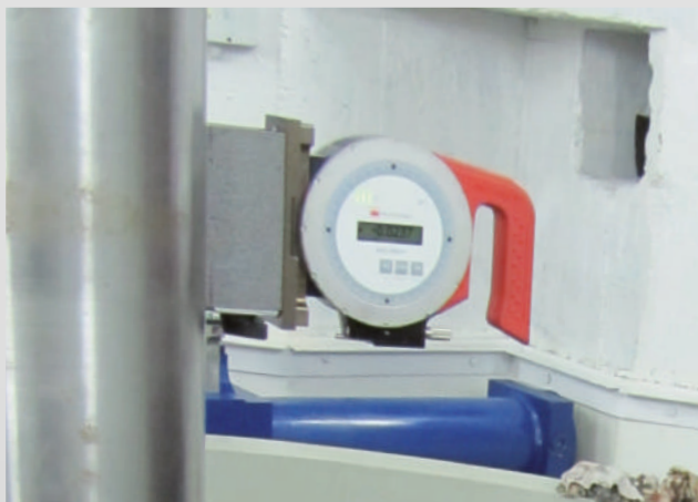
Plumbness measurement of a vertical shaft
