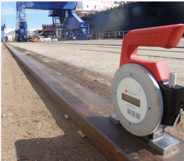
Straightness measurement of a port crane rail
